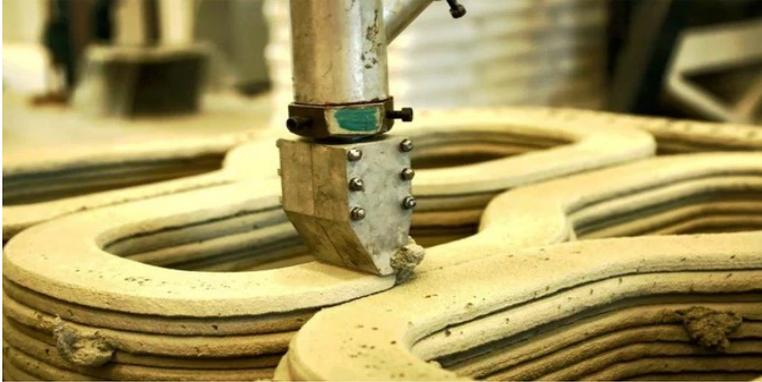
A new cyclist bridge completely 3D printed has just opened in the Netherlands. Designed and built by engineers from the Technical University of Eindhoven and the construction company BAM Infra, the bridge was printed in pieces from a concrete mixture and reinforced with steel cable, before being assembled and erected on-site.
