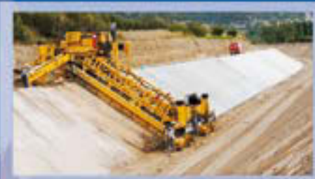
Beton Döşeme Teknolojisi (finisher) GOMACO The World wide Leader in Concrete Paving Technology
