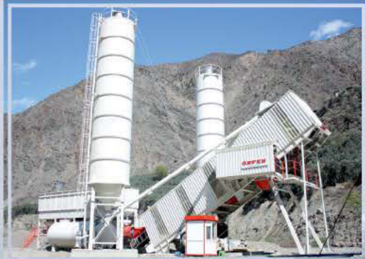
70 m 3 /saat MOBİL BETON SANTRALİ - ARTVİN / YUSUFELİ BARAJI
